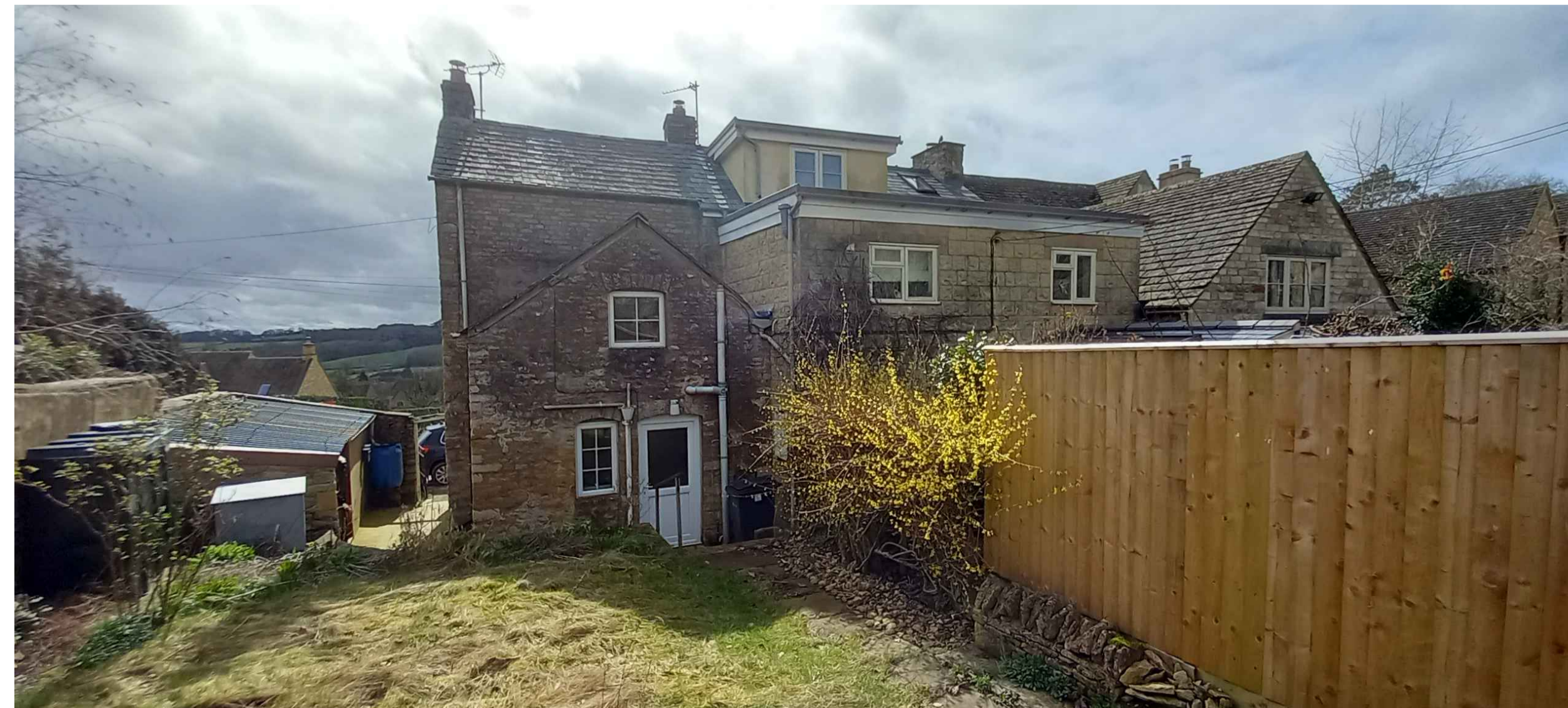
VALLEY VIEW - REAR PHOTOGRAPH
